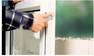
Depending on the fixing method, either screw in securing anchors in each window corner or drill holes in the side of the frame (corner distance approx. 15 cm).
