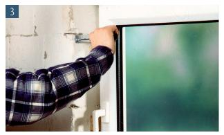
Remove the casement. Drill and screw through the wall anchor or the frame into the masonry. Reinsert the casement.
