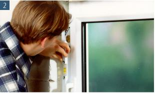
Place the window in the wall opening, align it with the spirit level and fix it in the corners with wedges. Then carefully perform a function check.
