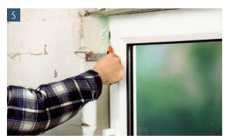
After hardening, cut off the excess installation foam with a sharp knife.
