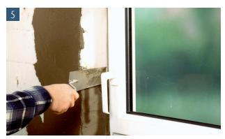
Cover joints vapour-tight inside and driving rain-tight and diffusion-open on the outside. Finally, clean the new window.
