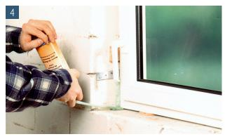
Insulate the cavities with non-pressing foam (frame foam).
