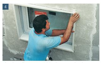
After the wall covering work has been completed, insert the assembled insulation connection profile into the groove left free by the removal of the formwork seal.
