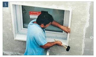
Fix by hammering into the groove (e.g. rubber mallet). Sealing between the insulation connection profile and the façade can be carried out with commercially available sealants (façade adhesives).
