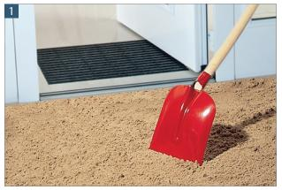
Prepare the substrate so that the upper edge of the ACO shoe scraper Vario is flush with the adjacent surface covering. (important for the following steps!)
