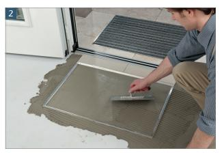
To create a flat support for the mat, apply tile adhesive evenly to the lower edge of the frame.
