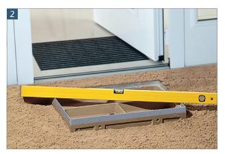
Place and align the floor tray of the shoe scraper on the substrate.
