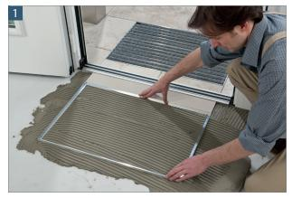
Place the angle frame on the prepared tile adhesive, align and press
